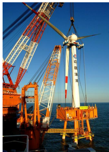
Figure 6: Bohai turbine installation
