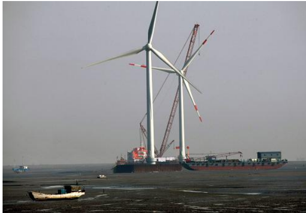
Figure 9: Longyuan Group erects first turbines in Intertidal zone at Rudong Intertidal project
